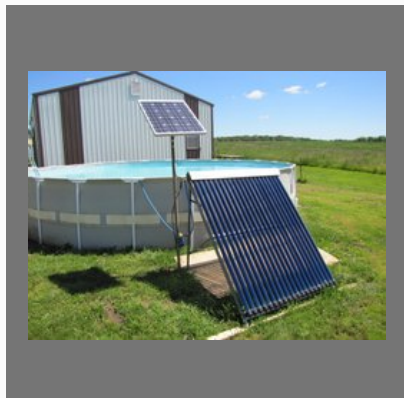
Solar Hot Water Heater
