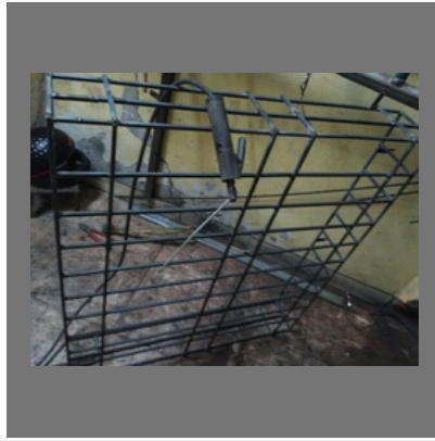
Window Grill Fabrication
