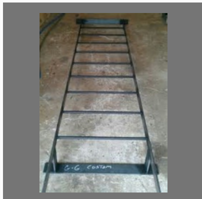
Steel Ladders Fabrication
