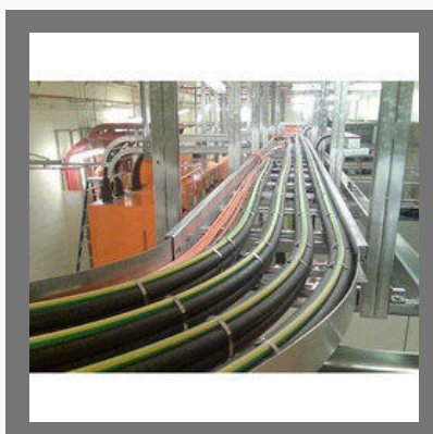
Cable Tray Installation Service
