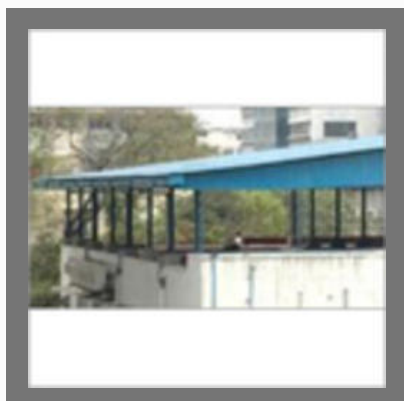
Roofing Installation Services
