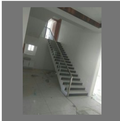
Stainless Steel Railing
