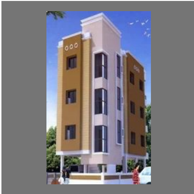
Apartment Construction Service
