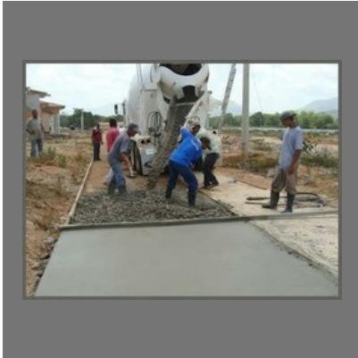
Rcc Roads Constroction
