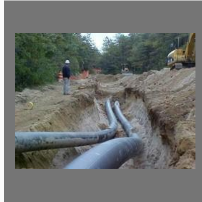
HDPE Pipe Installation
