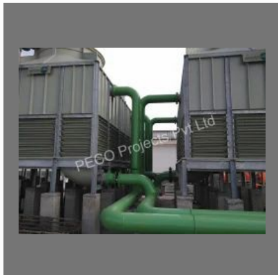
Cooling Water Piping Installation Service
