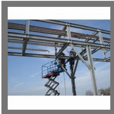
Pipe Rack Bridge Erection Service
