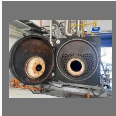
Boiler Annual Maintenance and Inspection
