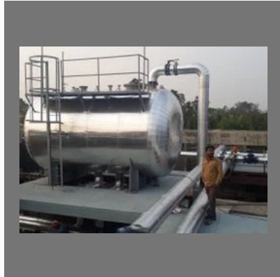
MS Storage Tank Fabrication
