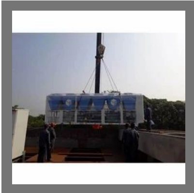
Chiller Erection Service
