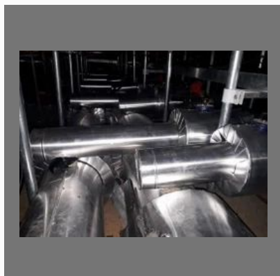
Low Side Piping Installation Service
