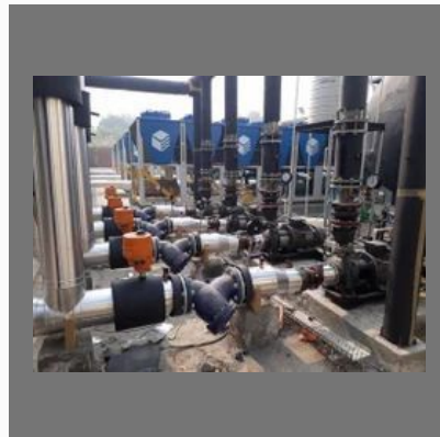
Data Center Piping Installation Service
