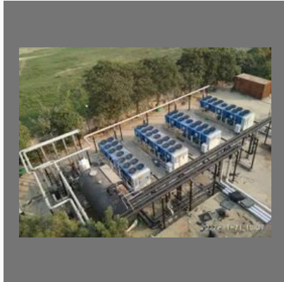
Chilled Water Piping
