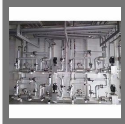
Pipe Skid Fabrication Service
