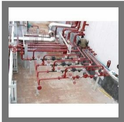
MS Piping Fabrication
