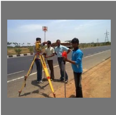
Road Survey Services
