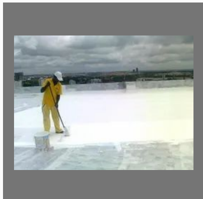
Building Waterproofing Service
