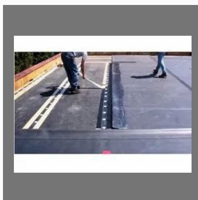
Roof Repairing Service
