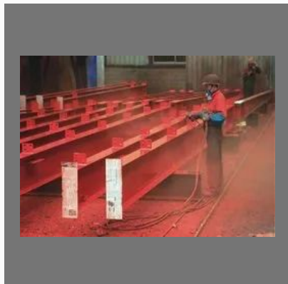
Spray Galvanizing Service
