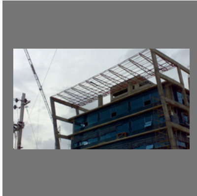
Glazing & Glass Works
