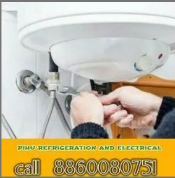
Gijar Repairing Service
