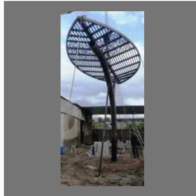
Mild Steel STRUCTURE
