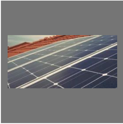
Solar Grid Tied System
