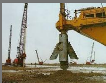
Under Reamed Piling Services
