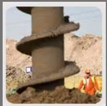
Bored Compaction Pile Service
