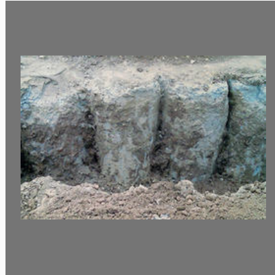
Touch Pile Service
