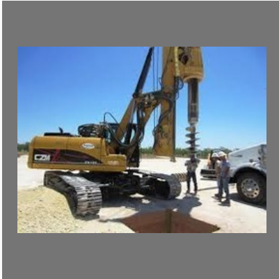
Pile Foundation Service
