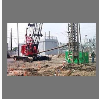
Machine Foundation Work
