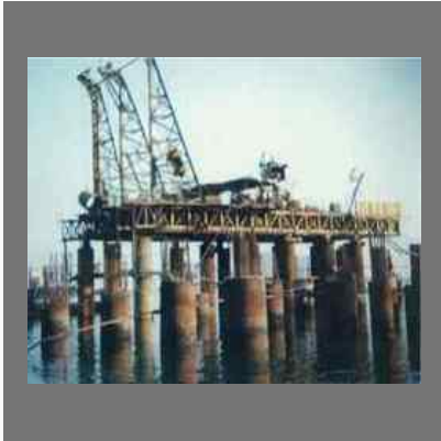
Marine And Off-shore Piling Services
