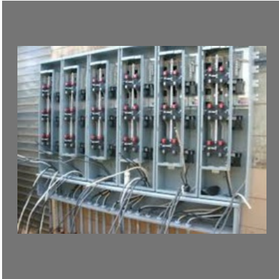
Commercial Electrical Works
