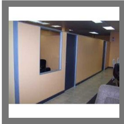
Cement Drywall Partition
