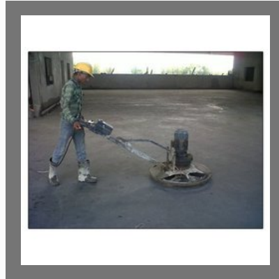
Tirmix Flooring Service
