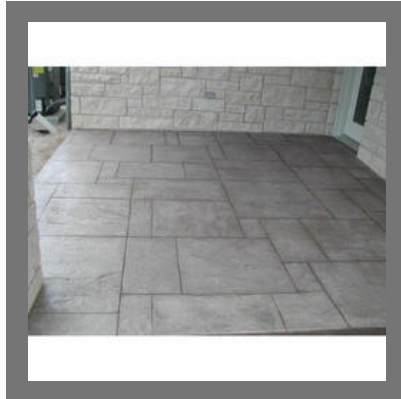
Stampcrete Pathway Flooring Service
