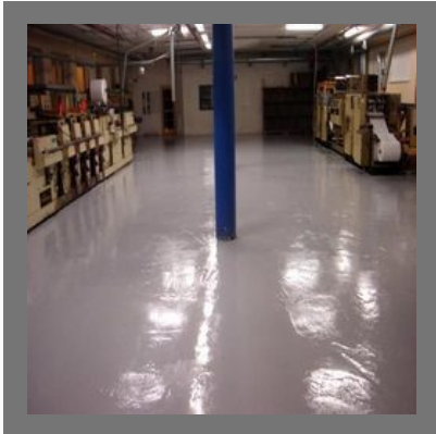
Water Based Floor Coating Service in Mumbai
