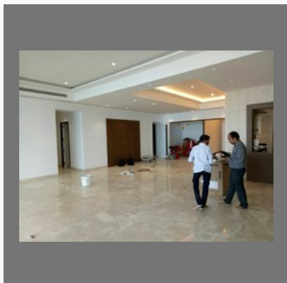
Gypsum P O P Ceiling Work
