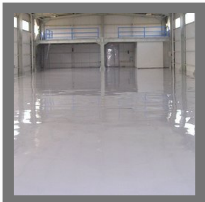
Self Leveling Epoxy Flooring
