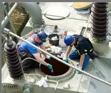
Tapchanger Inspections Repairs
