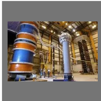
High Voltage Testing
