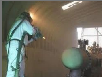
Sandblasting And Painting
