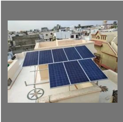
Solar System Installation Service
