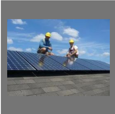
Solar Panel Installation Service
