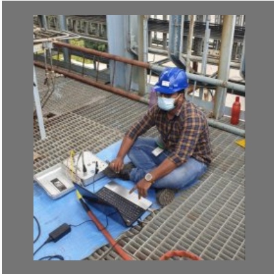
Online Safety Relief Valve Testing Service
