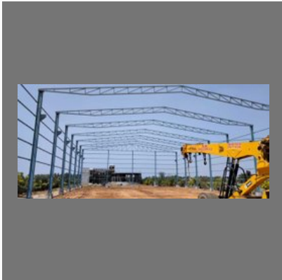
Prefabricated Structure Fabrication Service
