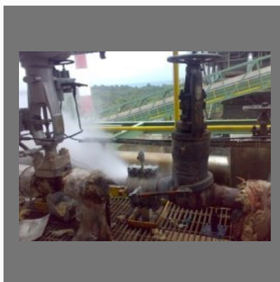
Online Leak Sealing Service
