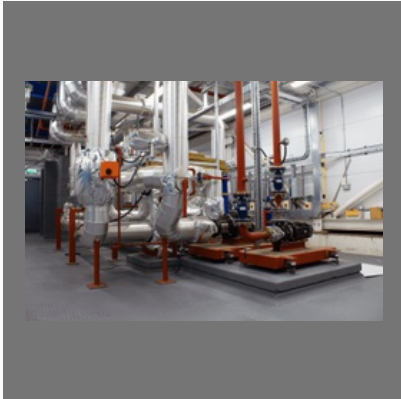
Industrial Pipe Fabrication Services
