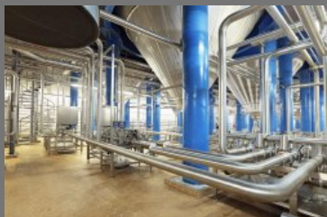
Industrial Pipeline Erection Service
