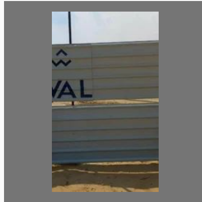
Tin Sheets Compound Wall
