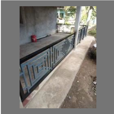
Mild Steel Balcony Railing
