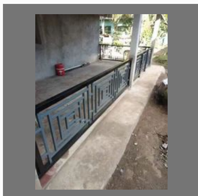
Mild Steel Balcony Railing
