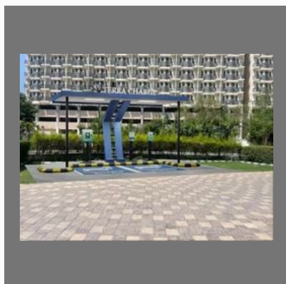
E V Charging Station Construction
