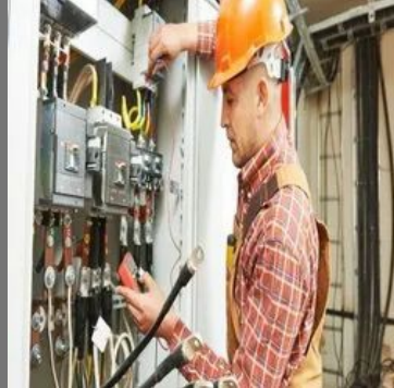
New Building Electrical Work
