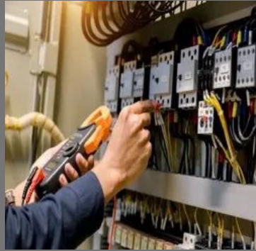
Industry Electrical Wiring Work
