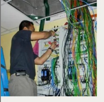
Residential Building Electrical Work
