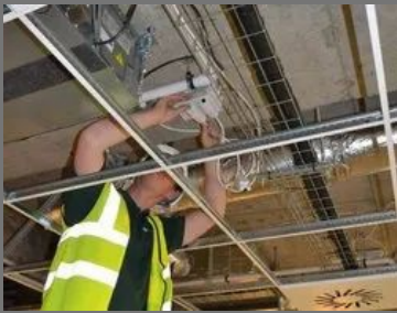
Commercial Buildings Cogeneration
