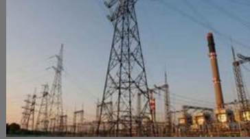
Contractors For Erection & Commisioning Of Power Plants
