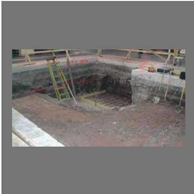
Industrial Foundation Structures Construction
