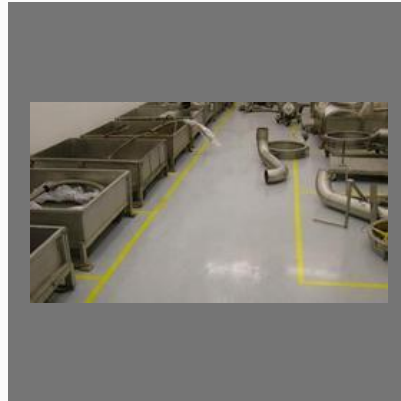
Industrial Flooring Construction
