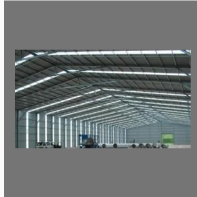
Industrial Shed Construction
