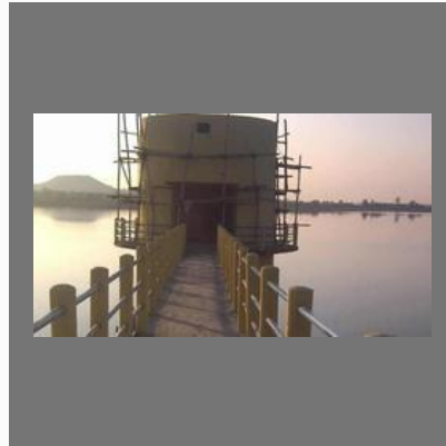
Repair Of Intake Wells
