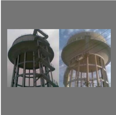
Overhead RCC Water Tanks Construction
