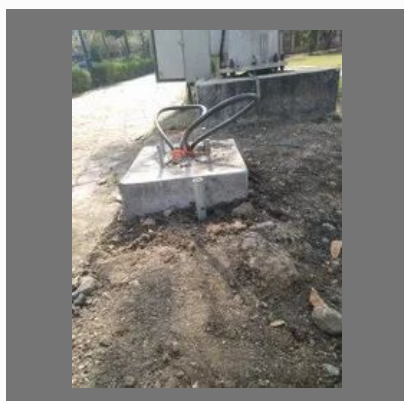
Electrical Construction Service nagpur
