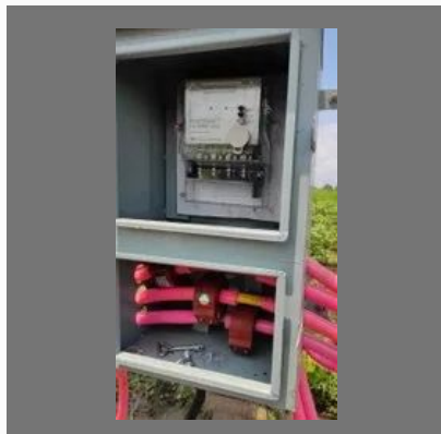
Paneling And Electrical Works
