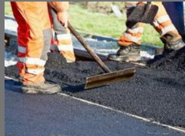
Civil Work Construction of Road
