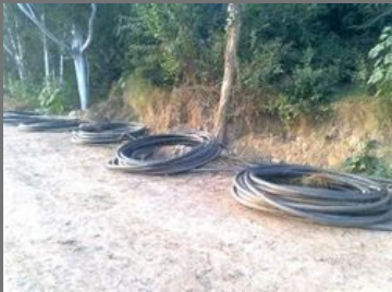
Cable Laying Work
