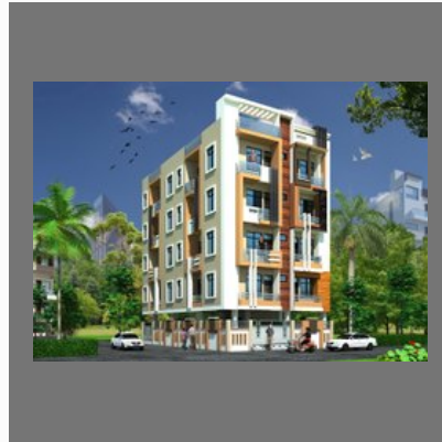
Commercial Construction Service
