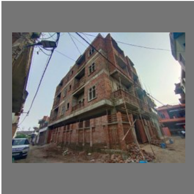
Civil Work Services
