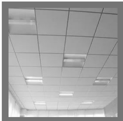
False Ceiling Installation Service
