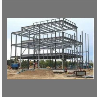
Pre Engineering Steel Building
