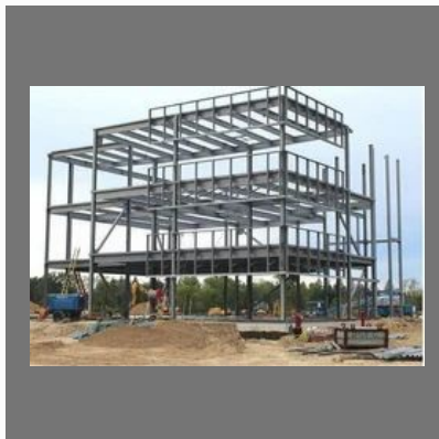
Pre Engineering Steel Building
