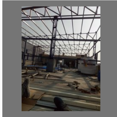
Prefabrication Building Service
