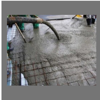
Small Loads Of Ready Mix Concrete
