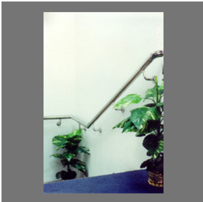
Stainless Steel Handrail
