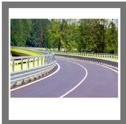
Metal Crash Barrier Systems
