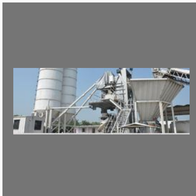
Cement Factory Construction Services
