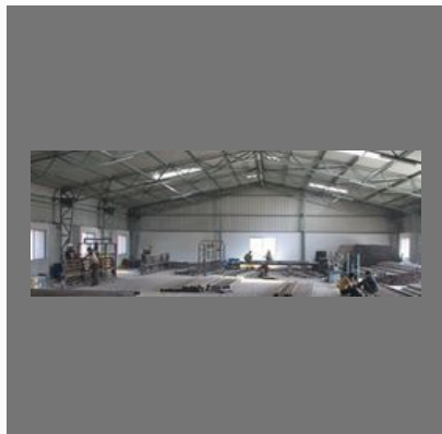
Factory Buildings Construction Services
