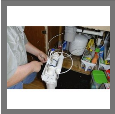
Water Purifier Installation Service
