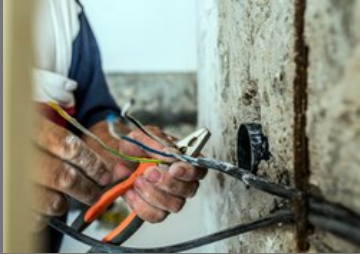
Wiring Contractor Service
