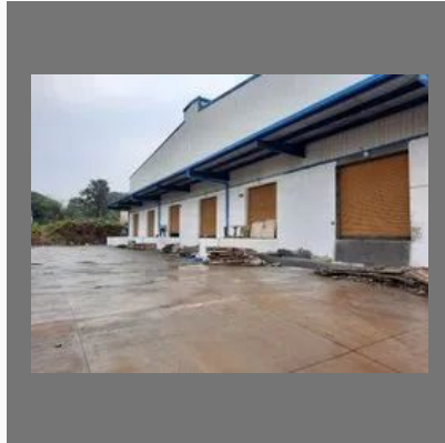
Industrial Concrete Flooring Service
