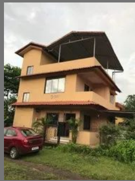
House Construction Service
