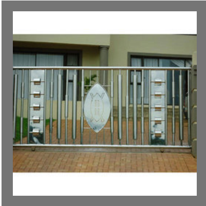
Stainless Steel Main Gate
