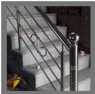
Stainless Steel Railing
