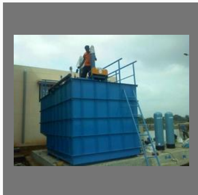
Sewage Treatment Plant Maintenance
