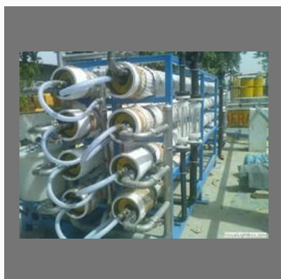
Effluent Treatment Plant Erection Services
