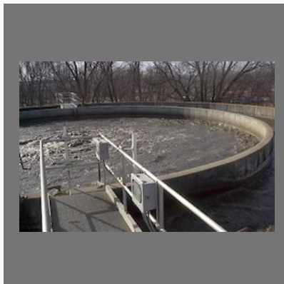
Water Treatment Plant Maintenance
