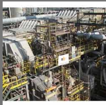
Revamping Sewerage Services
