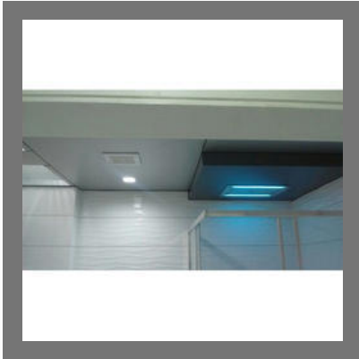
Bathroom False Ceiling Service
