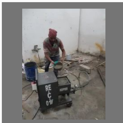
Basement Waterproofing Services Mumbai
