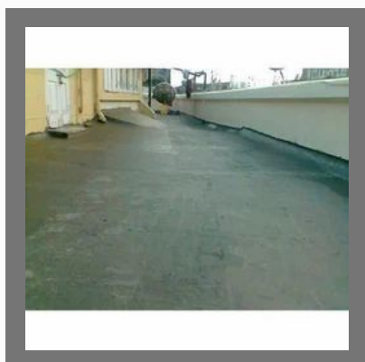
Membrane Waterproofing Service
