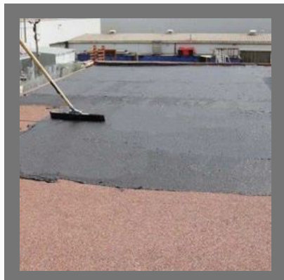
Bitumen Waterproof Coating
