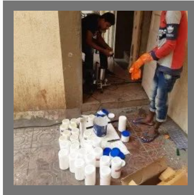
Pressure Grouting Service
