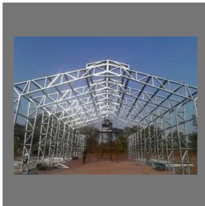
Mild Steel Factory Roofing Structure
