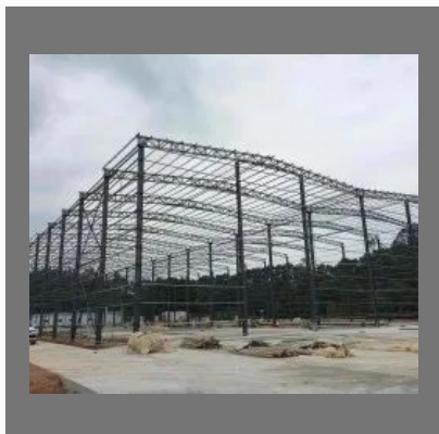
Mild Steel Godown Roofing Structure
