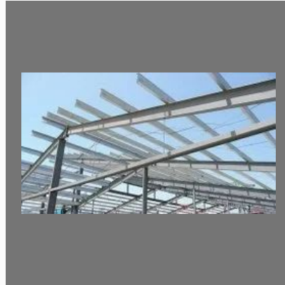
Godown Structural Fabrication Work
