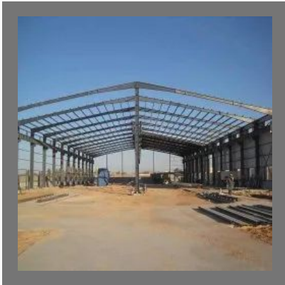
Warehouse Steel Roofing Fabrication Work
