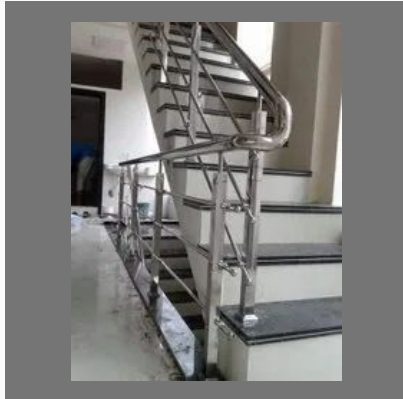
Stainless Steel Staircase Railing
