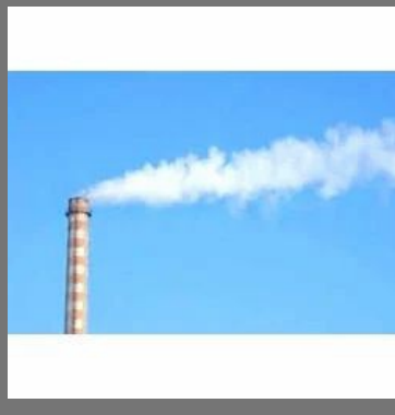
Industrial Smoke Chimneys
