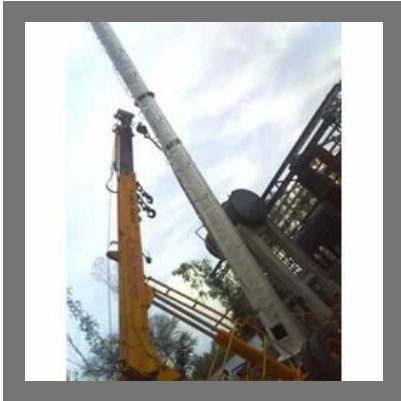
Rope Supported Chimneys
