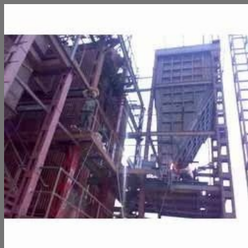
Boiler Erection Services
