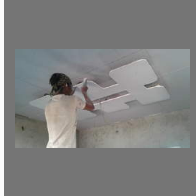
POP Ceiling Work
