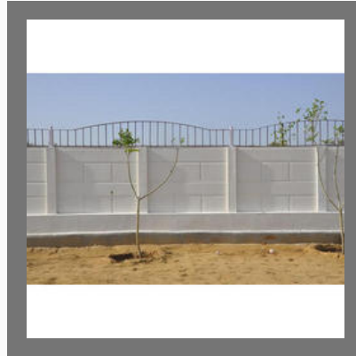
RCC Precast Boundary Wall
