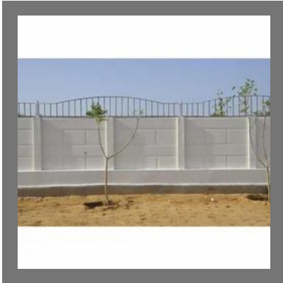
RCC Precast Boundary Wall
