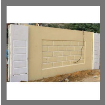
Concrete Compound Wall
