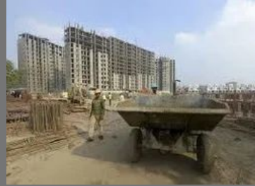
Apartments Construction Service
