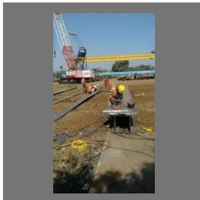
Pre Engineered Building
