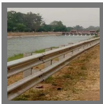
Single Sided Double Beam Crash Barrier
