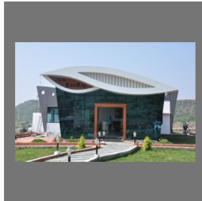
Glass Glazing Work
