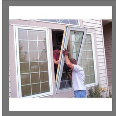
UPVC Window Installation Service
