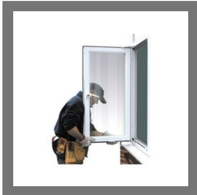
PVC Window Installation Service
