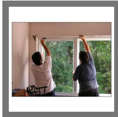
Aluminium Window Installation Service
