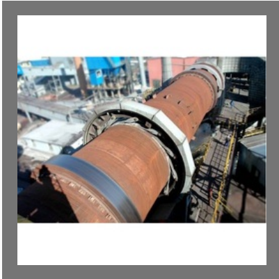
Rotary Kiln Calciner
