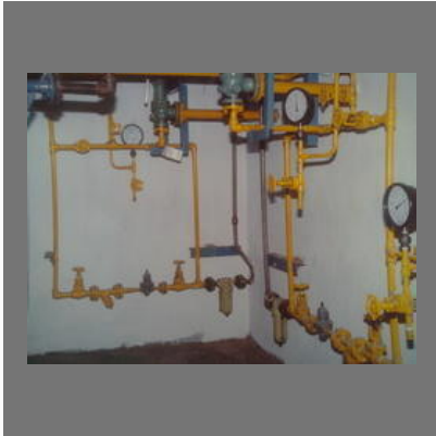
Utility Piping Fabrication Service
