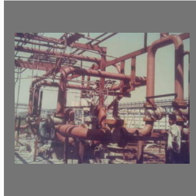
Piping Fabrication Service
